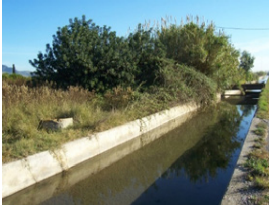
Figure 27: Forn de Vidre Mill Elaborated by the authors.
