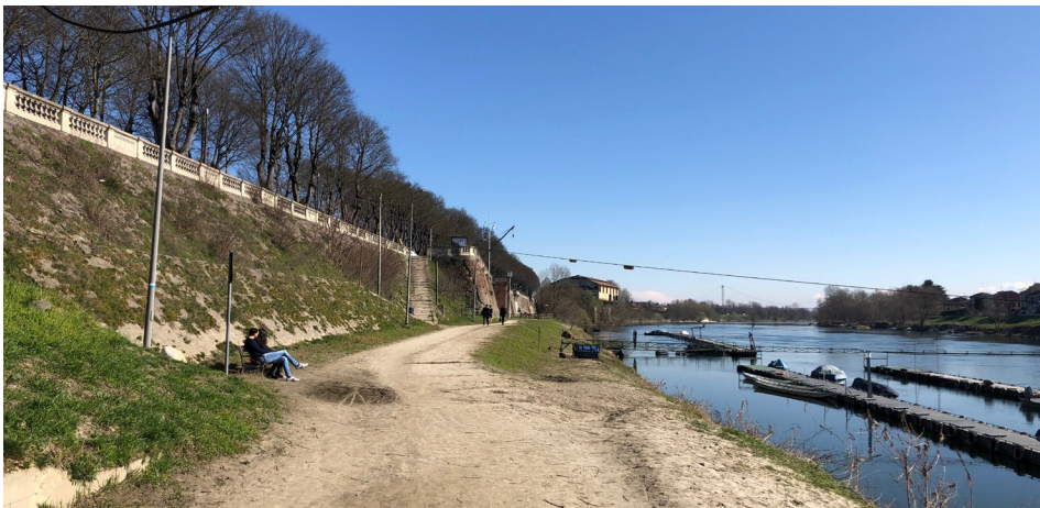
Figure 19 – Ticino embankment, Pavia Italy Fonte: Lorenzo Quaglini, Pavia University
