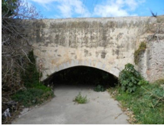
Figure 14: Barranquet Aqueduct Elaborated by the authors.
