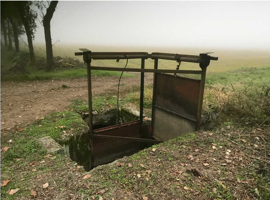
Figure 27 – Water intake, Pavia – Fonte : Silvia La Placa, Pavia University
