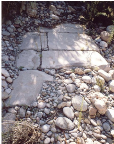
Figure 16: Castelló/Almassora New Weir Elaborated by the authors.
