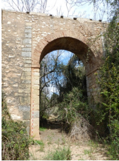
Figure 11: Barranc del Malvestit Aqueduct Elaborated by the authors.
