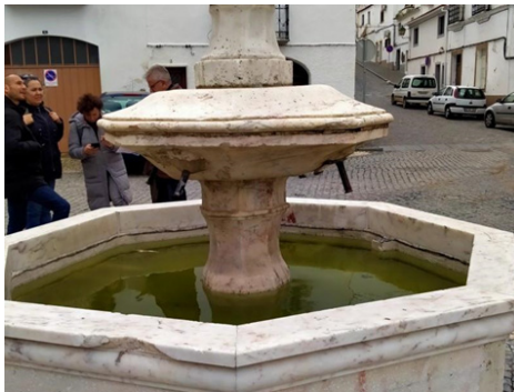
Figure 10: Fonte do Largo do Barata. Current status Elaborated by the authors.
