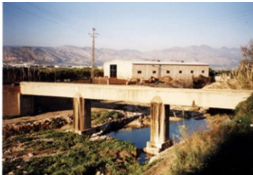
Figure 9: Aqueduct Sec River Elaborated by the authors.
