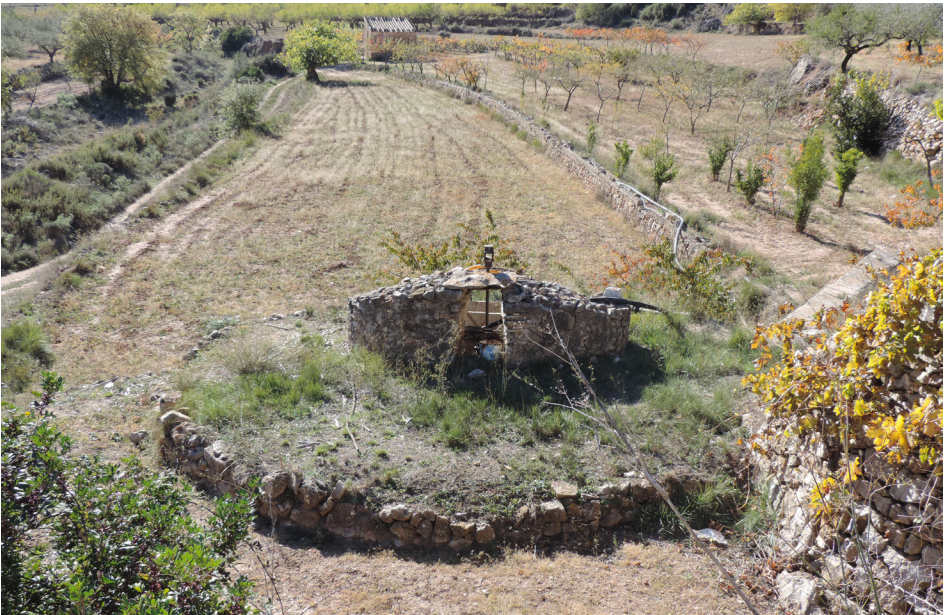
Figure 4 – Noria in Castellón de la Plana, Spain Source: Pablo Altaba Tena, Uji University
