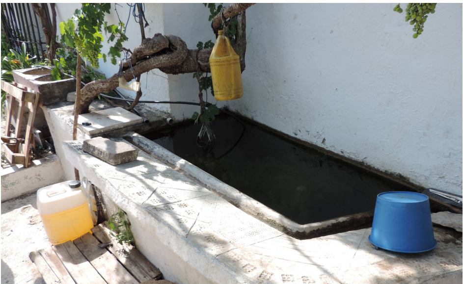
Figure 17 – Laundry, Spain Source: Pablo Altaba Tena, Uji University
